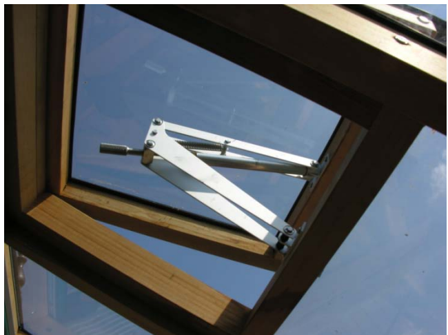
Above picture shows a triple spring autovent
